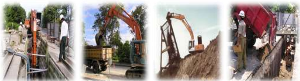
Gambar 2.6 Pelaksanaan Prinsip "Clean Construction"
